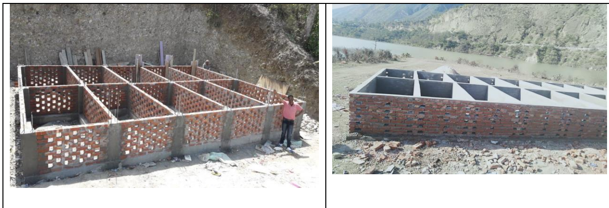
Aerobic honeycomb composting pit model
